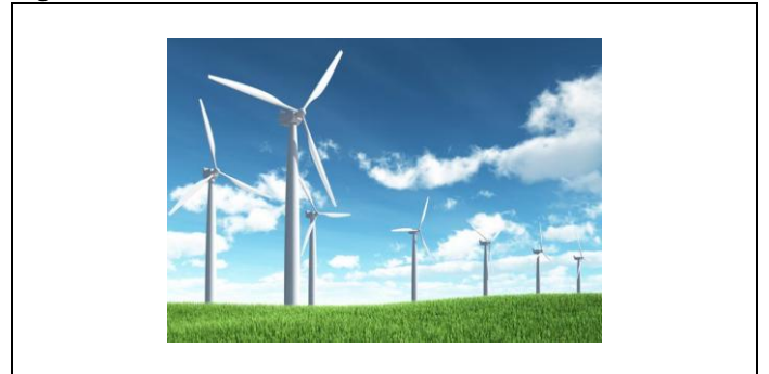
Figure 6. Wind Turbine Farm
