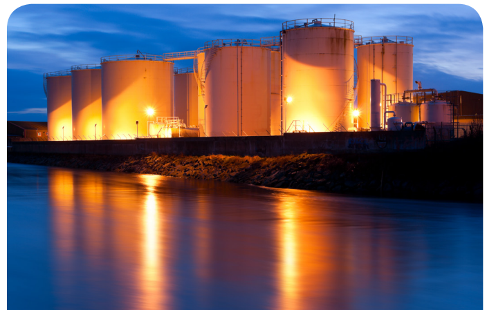
Large, industrial oil tanks in a remote location.
