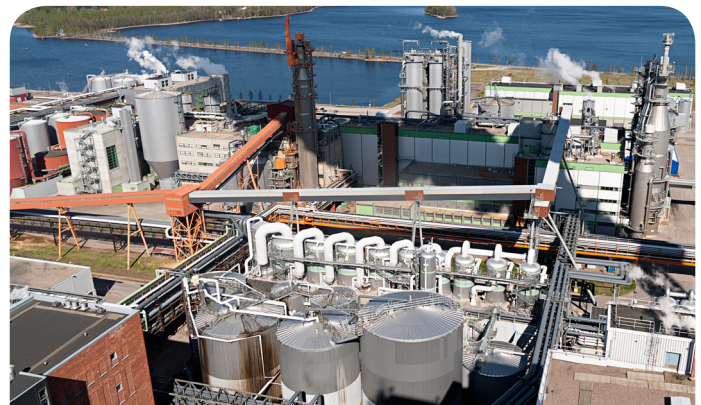
Paper production workshops throughout a large pulp and paper mill.
